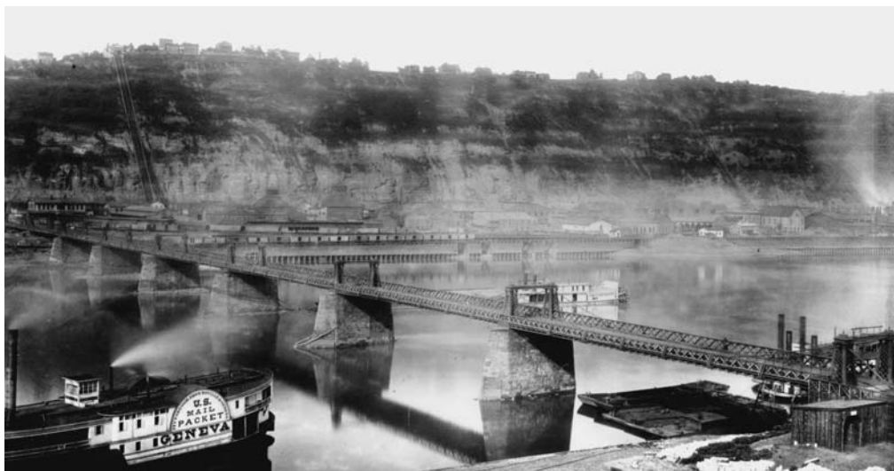
Figure 7. The Roebling wire-rope suspension bridge across the Monongahela River at Smithfield Street in Pittsburgh, built 1845-46. From Photo Collection, Carnegie Library of Pittsburgh, by permission., file #P-3109.(no date) (no photographer name).
